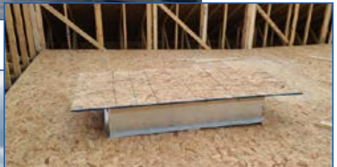
One of the new roof top unit (RTU) curbs for the heating/AC units on the admin building roof; they also help level the units on the slightly-pitched roof
