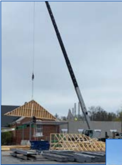
Wooden roof trusses being lifted into place over the porte cochere
