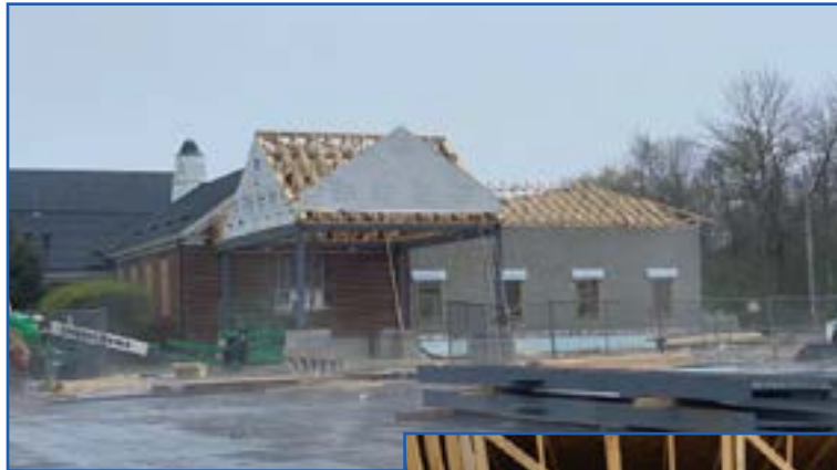
Roof trusses are in place
