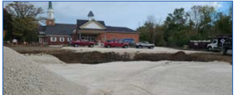
The layers of a parking area are important to maintain a level surface as well as proper drainage.
